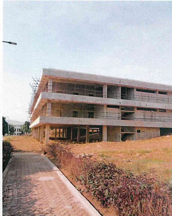
School of Mining and Geology Building
